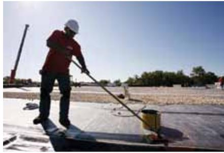
Maintenance crews can easily fail to notice these situations, allowing water to enter the roof system damaging insulation, roof decking and interior spaces. If the existing roof system includes a vapor barrier or has a second roof installed, water that enters the roof system might be trapped, damaging system components even though it is not leaking into the facility.
