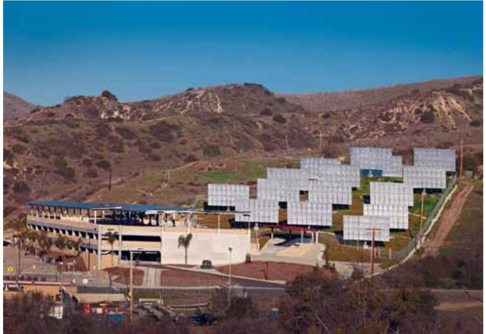
Pictured is the concentrated photovoltaic array that helps power the new recruit barracks complex.
